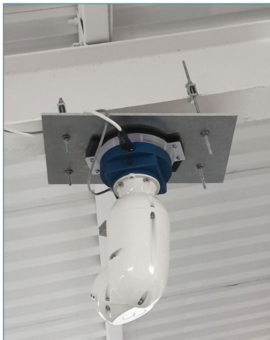
Figure 24 FiX1 installation on a customised bracket
